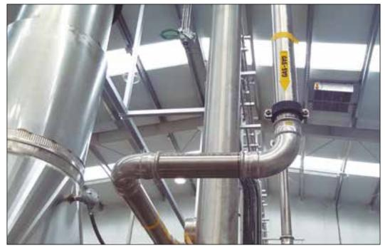
Pressing systems for natural gasand LPG installations made of Stainless Steel.
